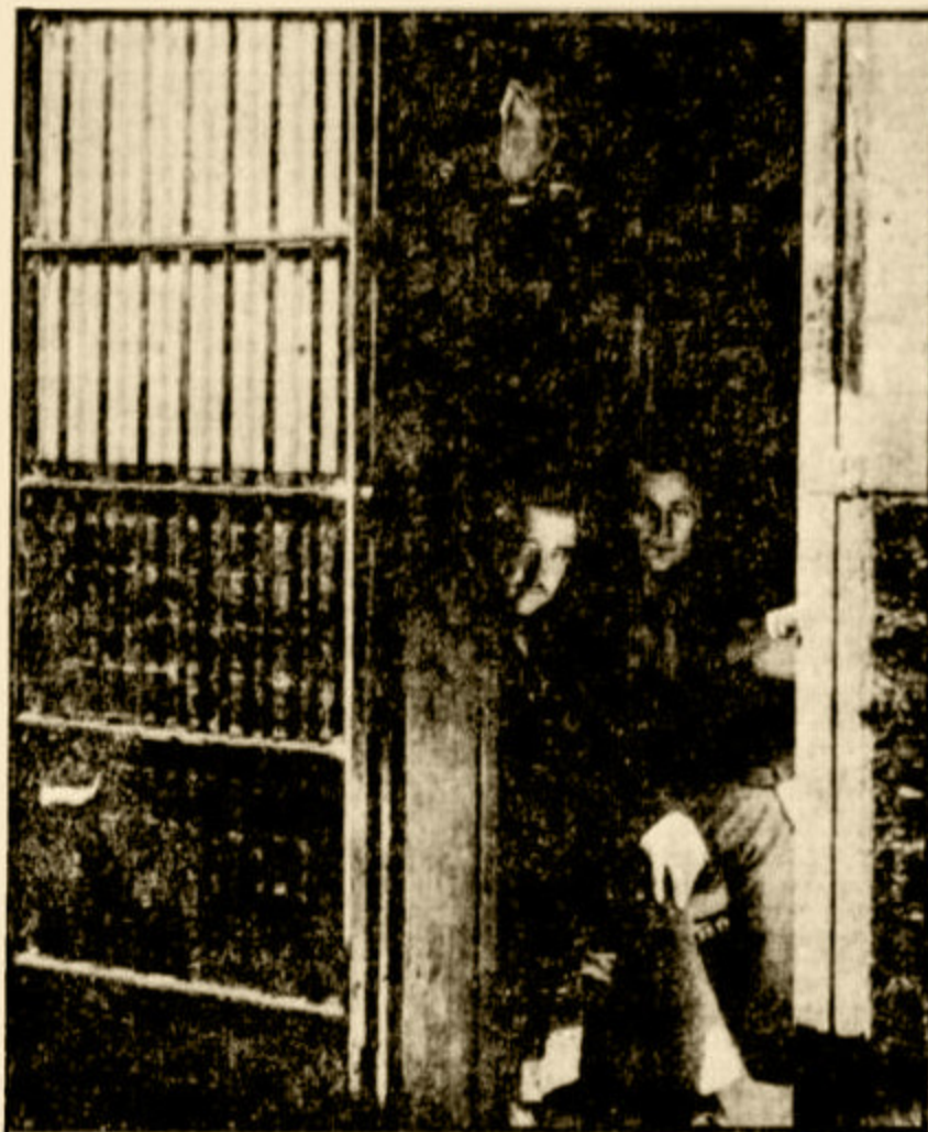
Narrow Cells at Workhouse.
